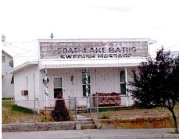
Building at the west end of Main Ave. Paint peels back to
