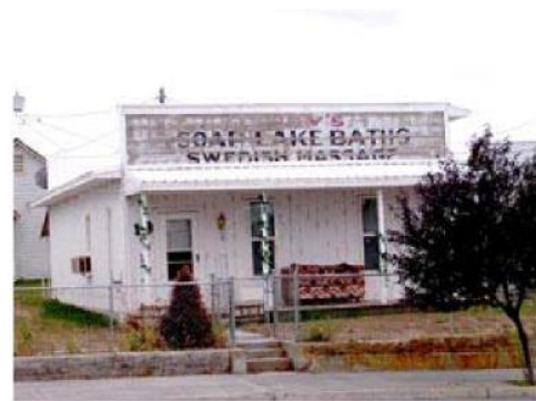
Building at the west end of Main Ave. Paint peels back to reveal interesting historic cues.
