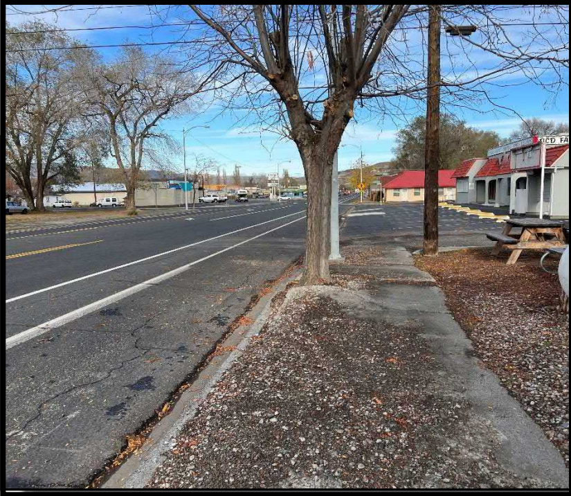
Daisy Street 3 rd Ave SE – looking North To be replaced!
