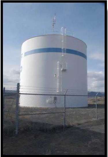
East Reservoir (Welded Steel)
