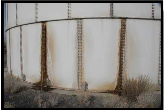
West Reservoir (Bolted Steel)
