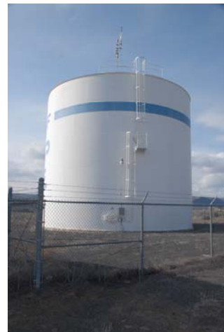
500,000 gal Welded Steel East Reservoir
